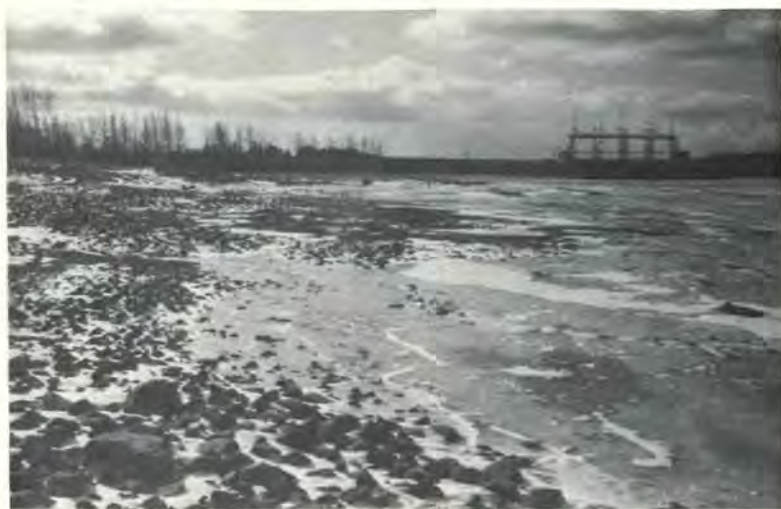
FIG. 7. Shand Dam, an earthfill-gravity dam, and Belwood Reservoir, on the Grand River, near Guelph, Ont., showing the drawdown zone (photo by R. M. Baxter).
